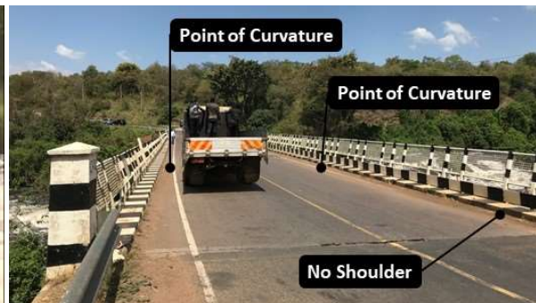
Lack of Shoulder Width in Curve Section
