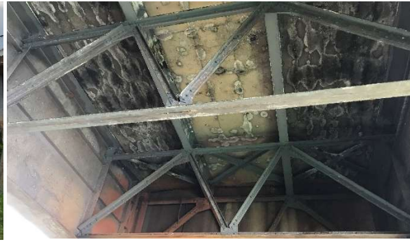
Deterioration of Slab, Corrosion of Steel Girder
