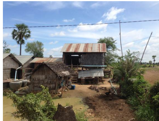
Photo4-4 : A private house. Pipes are installed from the roof to the water pot so that rainwater can be collected in the house on the left side (July 2017)
