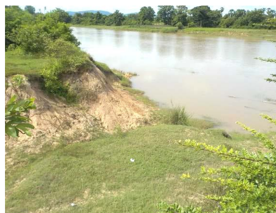
Photo2-4 : Drainage point from new WTP to Pursat River (Aug. 2017)
