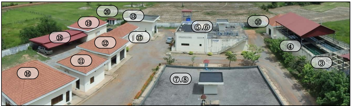
Figure 1-4-12 Overview of the Existing WTP from an Elevated Tank
