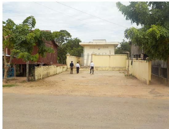
Photo1-2 : Existing Intake Pump Facility (June 2017)
