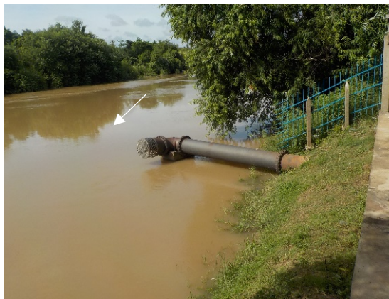
Photo1-1 : Existing Intake (June 2017)
