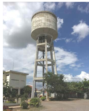
Photo1-6 : Existing Elevated Water Tank (June 2017)
