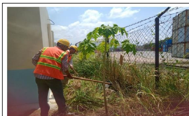
Photo 1: Clearance of grass and site in the Temporary Yard in April 2024
