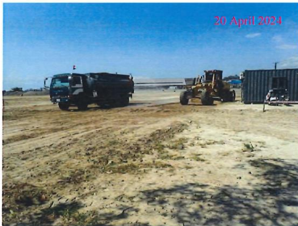
Photo 5: Grading, Compaction, and Watering at Temporary Yard in April 2024
