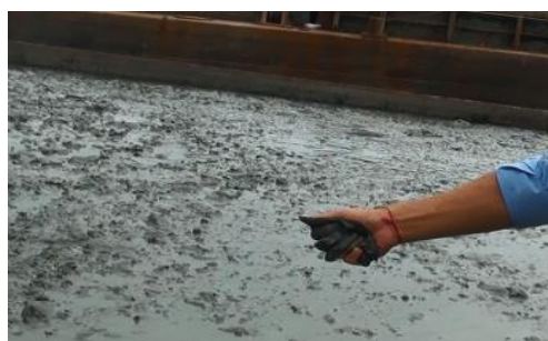
Figure 4-14: Dredged Soil in MPT
