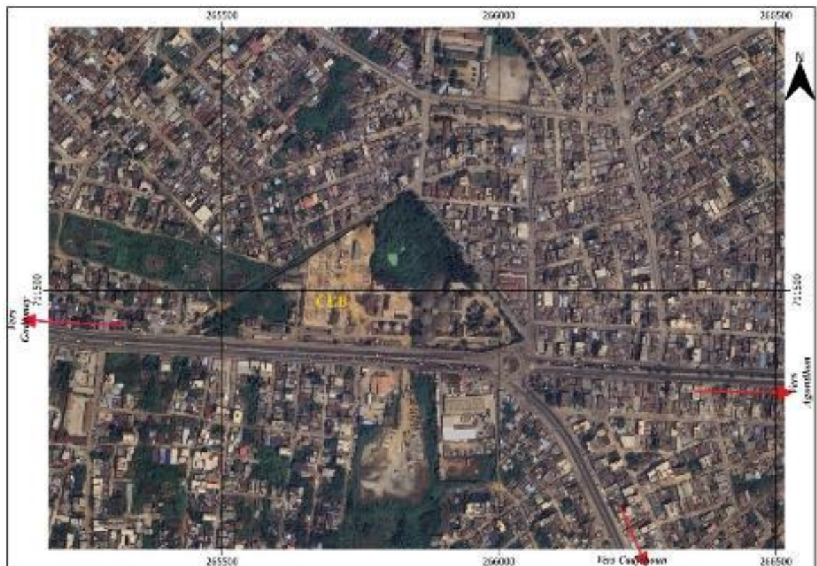
Figure: Overall view of the project area
