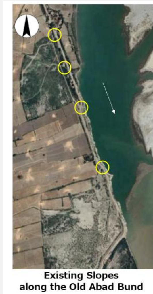
Figure 3.4: Existing Slopes at the Bund
