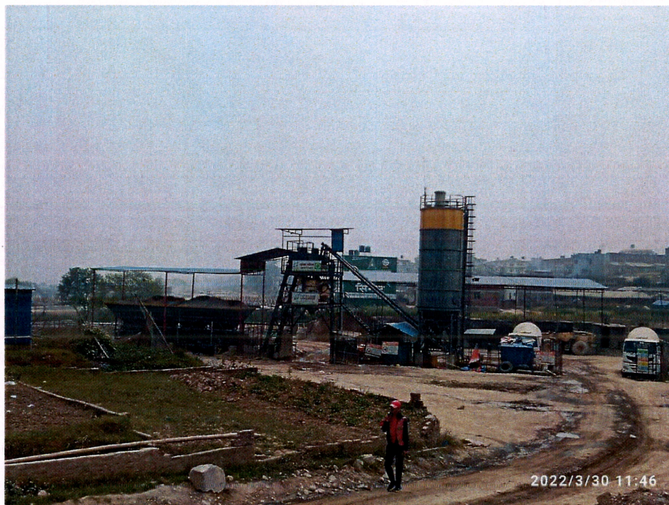
Figure 7-1: Batching Plant Site
