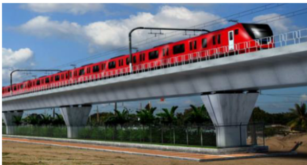
Figure 1-7 Cast in-situ/pre-cast segmental box girder sample illustration
