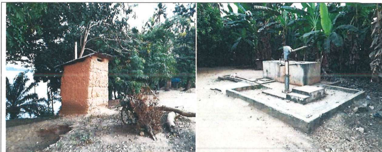
Photograph 2- 2: A household toilet facility at Volivo
