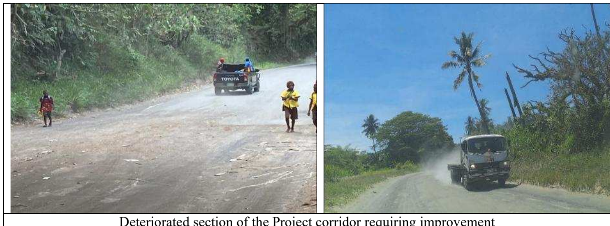
Deteriorated section of the Project corridor requiring improvement
