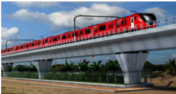
Figure 1-7 Cast in-situ/pre-cast segmental box girder sample illustration
