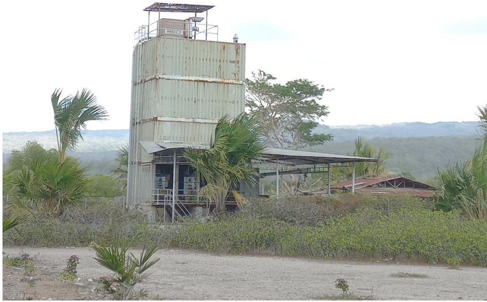
Figure 3 A photograph of the abandoned cement factory within the proposed project area in Carabela
