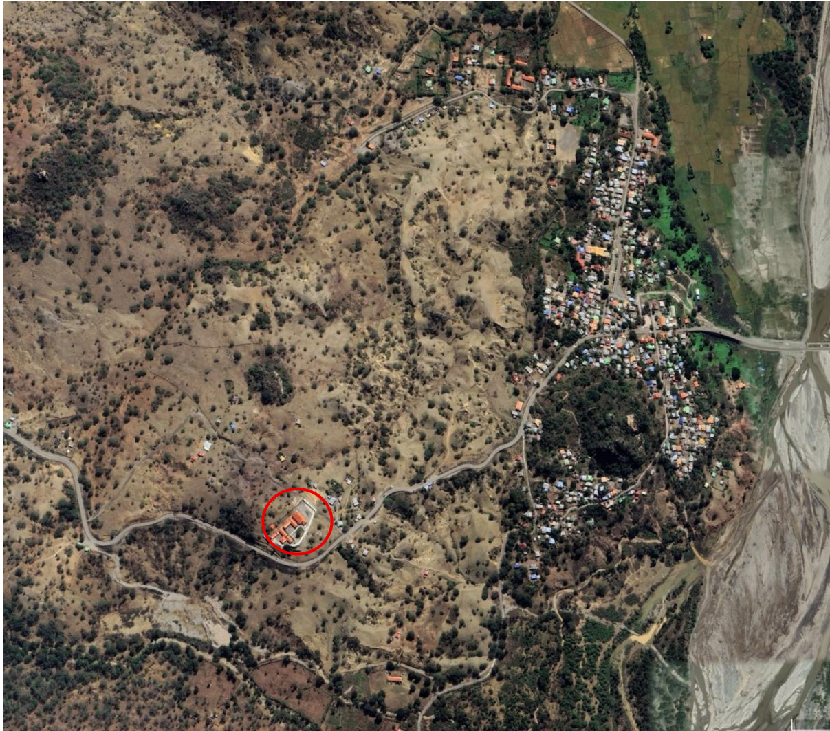
Figure 4-4 Public Water Supply – Administrative Building and Water Tank
