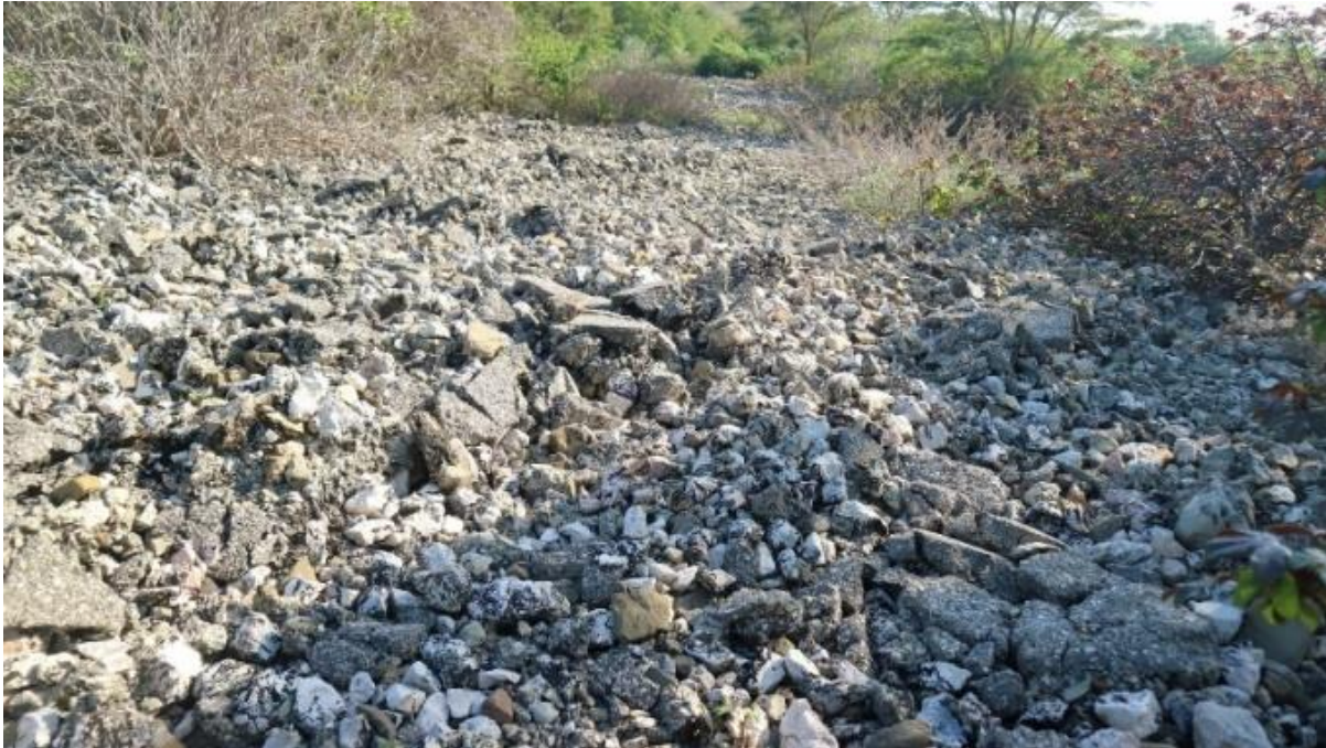
Asphalt dump on the project site
