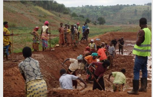
Community work for the construction of night storage (Nyabuyogera Site)
