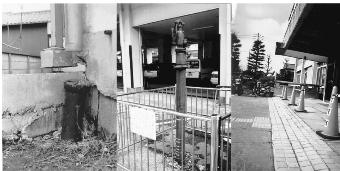
Rising of a Building in Urayasu City, Chiba Prefecture
