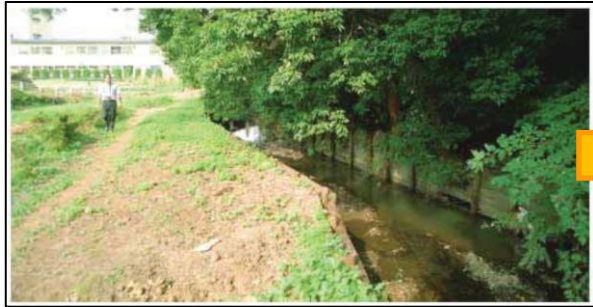
Before construction: plank hurdle revetment
