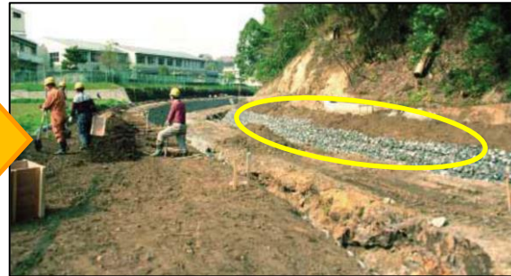
Renovation: Gabion revetment
