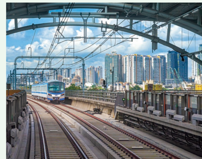
Ho Chi Minh City Urban Metro Line No.1 commenced operation, including the first underground section in Vietnam
