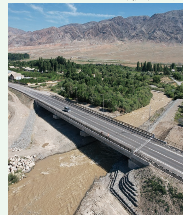
The rebuilt Urmural River Bridge (Sakura Bridge) in the Kyrgyz Republic, July 2024
