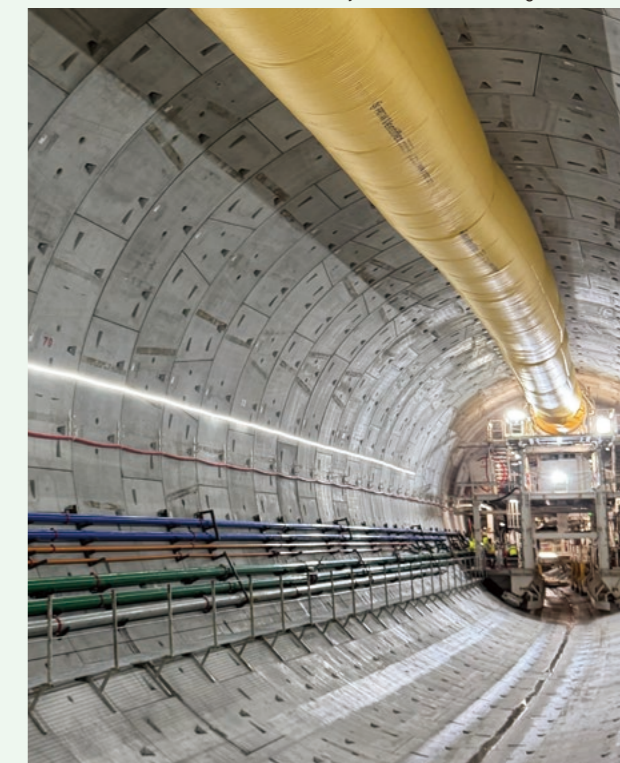
Site in Panama where subway shield tunnel drilling is underway
