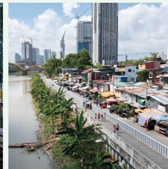
The levees in Metro Manila, the Philippines, constructed with JICA's cooperation
