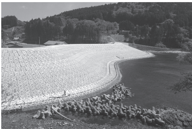
Figure 10-11: Seawall built after the disaster
