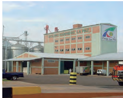
The completed flour mill. Source: JICA Paraguay Office
