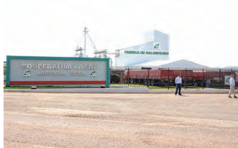
The feed factory.
