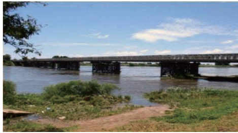
Existing “temporary” bridge.
