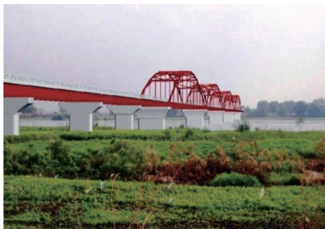
Image of completion of “Dream Bridge”.
