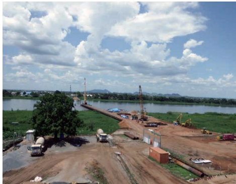
View of construction of “Dream Bridge”.
