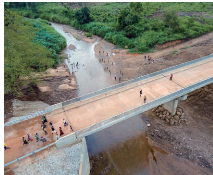
Aerial view of the completed Nyala Bridge Photograph: UNOPS
