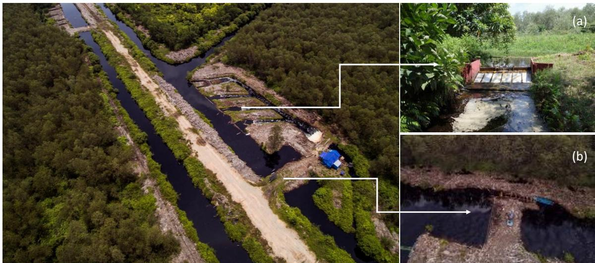
Fig. 9. Peat dam with “comb bypass” design: Spillways structure (a) and Peat dam (b)
