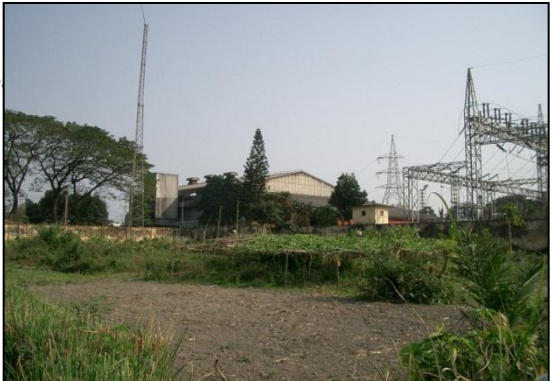
Existing Bheramara power plant seen from the construction site
