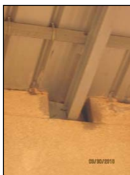
Photo 3 Narrow gap observed between the joist and the wall (Konni Department, Tahoua Region)
