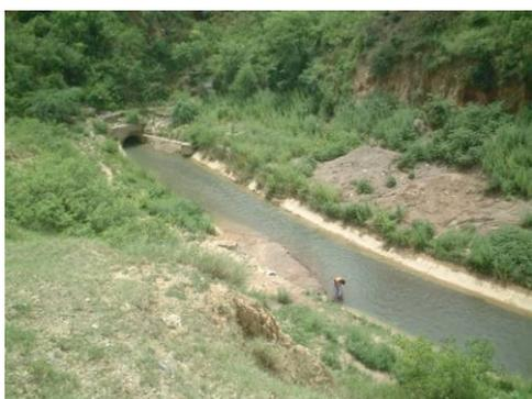
Figure 3: Silt in the canal
