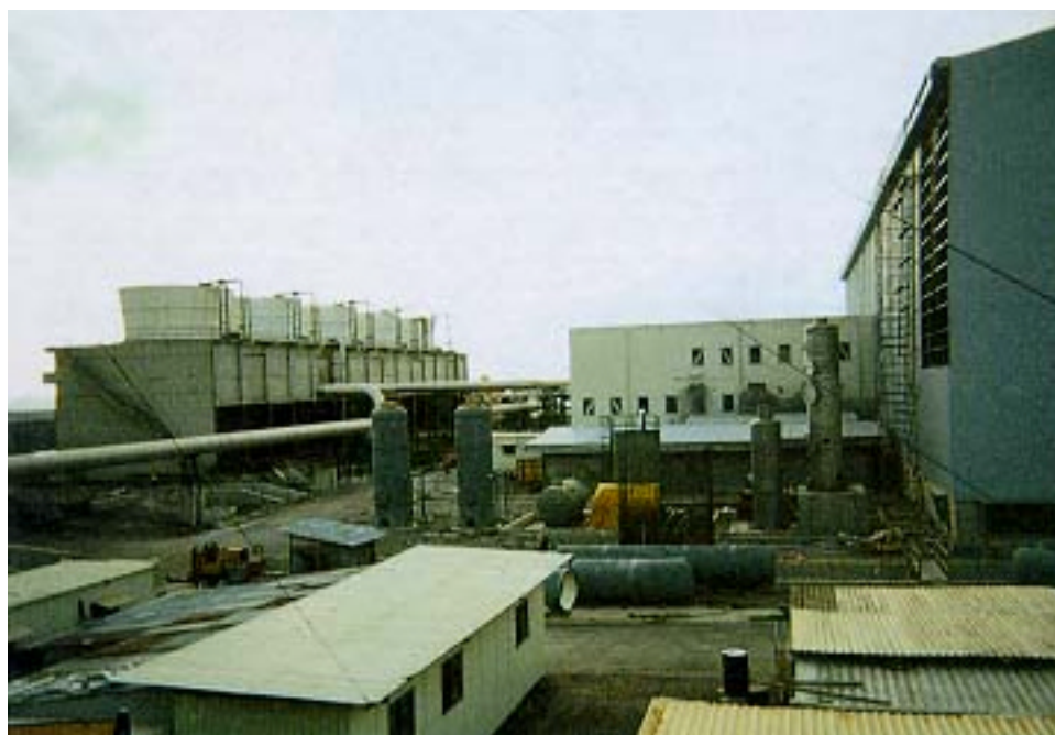
Construction of 2nd Plant
