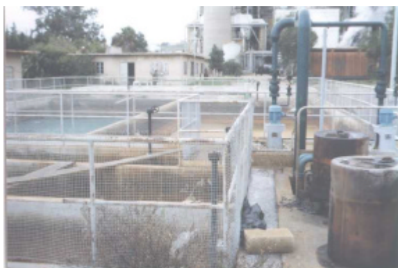
Household sewage water treatment tanks
