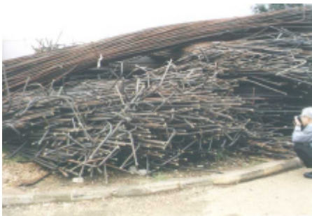
Stack of 11,780 replaced tubes, on plant premises
