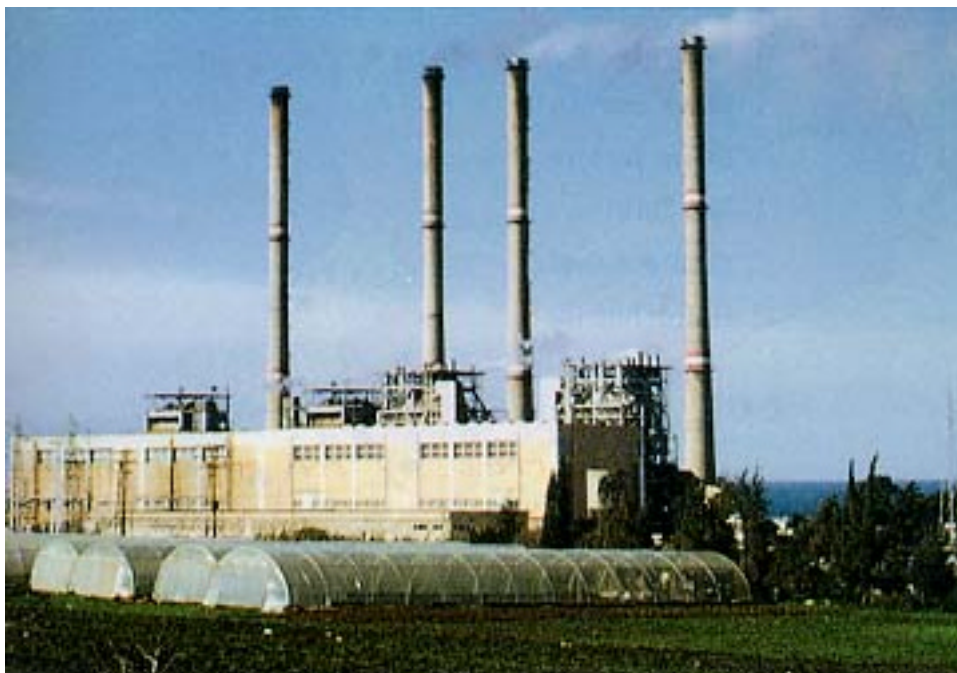
Distant view of Baniyas Power Station
