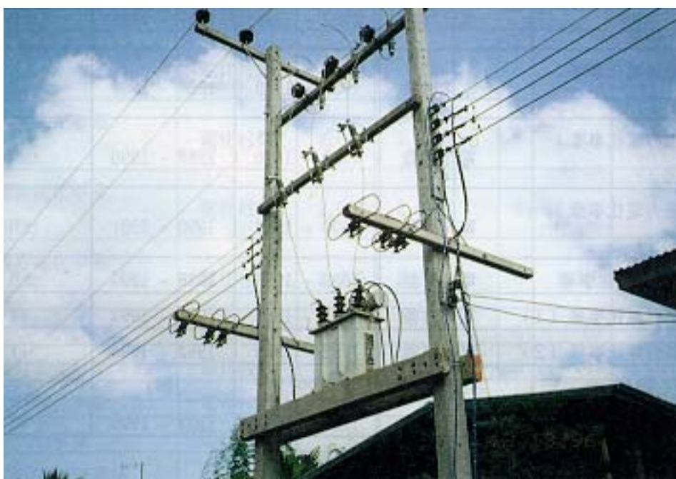
Pole Mounted Transformer for Distribution Restricted to the allowable strength of the electric pole, the large size transformer is mounted on a H-shaped structure as show in the picture. (Sakhon Nakhon, Bang Bon No.5)
