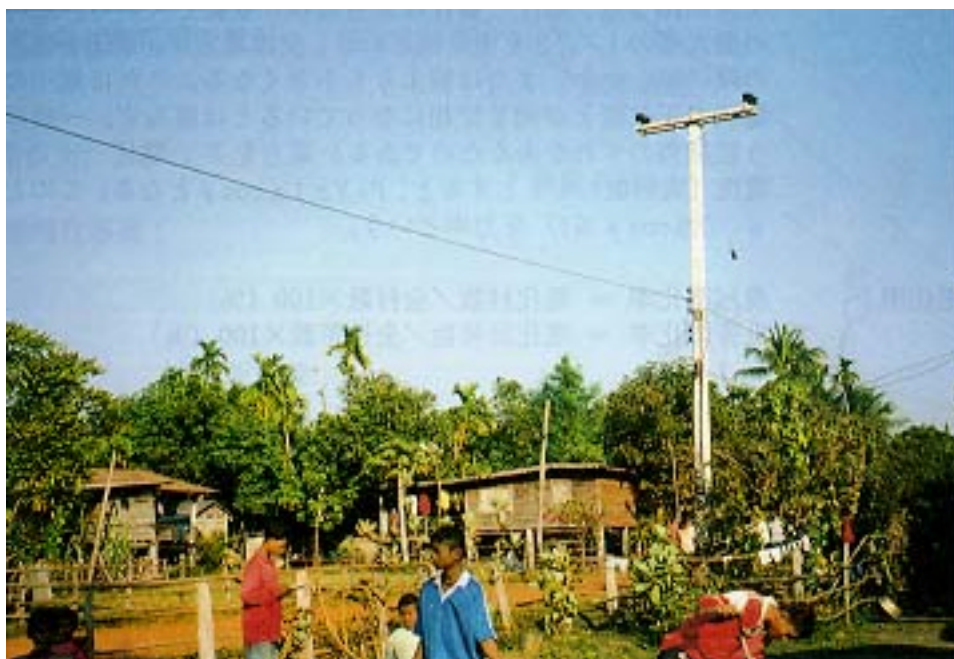
Distribution Line in the Village Upper level is High - voltage distribution line, lower level is Low - voltage distribution line. (Sakhon Nakhon, Bannalom)
