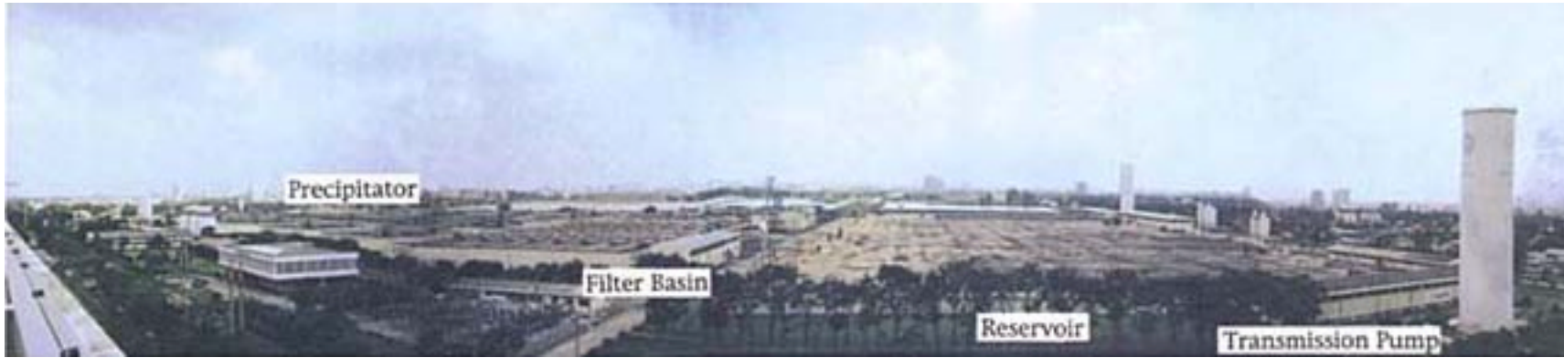
Over All Picture of Bang Ken Water Treatment Plant
