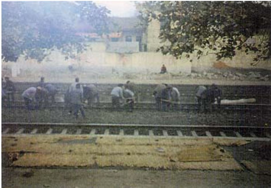
Manual Maintenance work of the Tracks (between Xian-Baoji)
