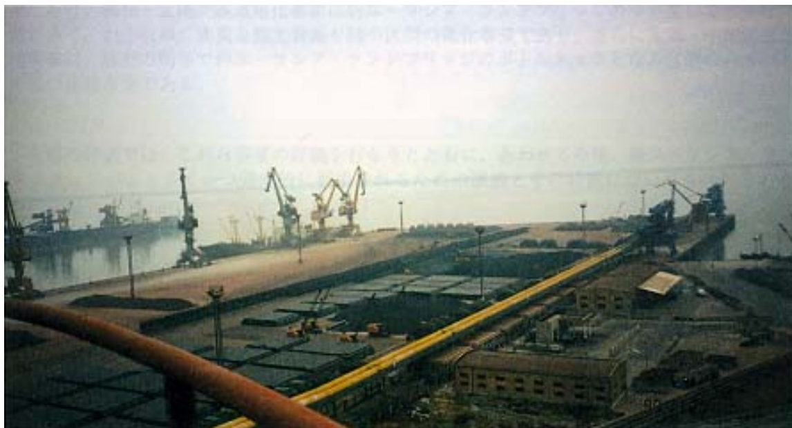
Overview of Project Site in Lianyungang Port The yellow pipes crossing the center of the photo are the pipes connecting Cereal berth and silos.
