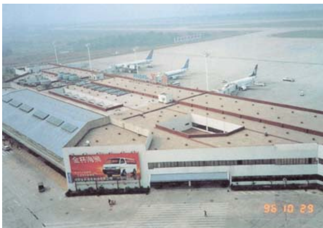
General Outlook of Passenger Terminal Apron (From Control Tower)
