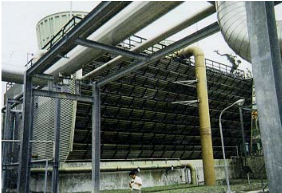
Cooling Tower at Generation Plant
