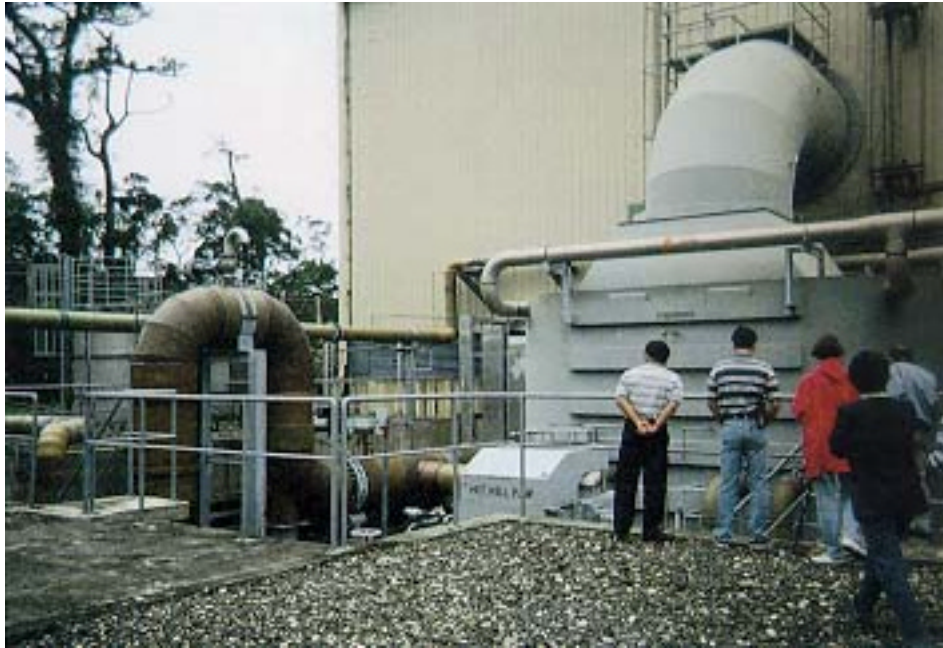
Condenser at Generation Plant
