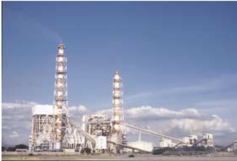
Calaca Coal-fired Thermal Power Plant (a complete view)
