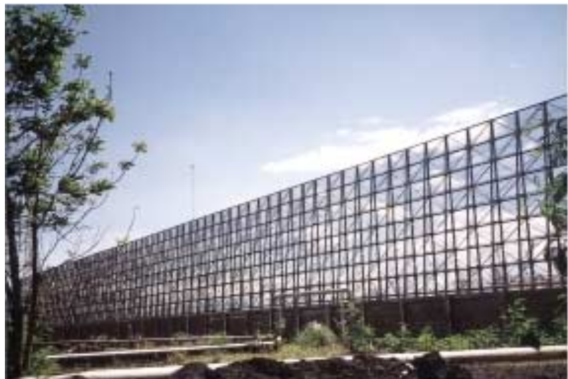
20m-high Windbreak Fence construction at the east and west side of the coal stockyard (one component of "Calaca I Coal-fired Thermal Power Plant Environmental Improvement Project")
