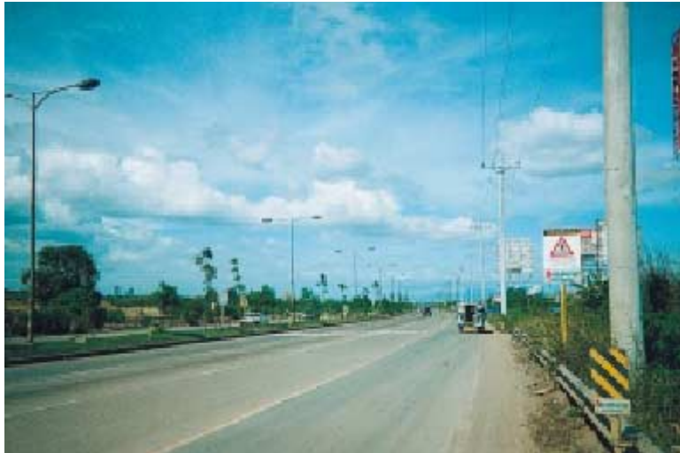
8-lane road with a median strip of Metro Manila Circumferential Road No.5 (Quezon City)
