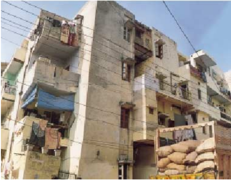
Houses for low income households financed by Housing Finance Company (Suburb of Delhi City)
