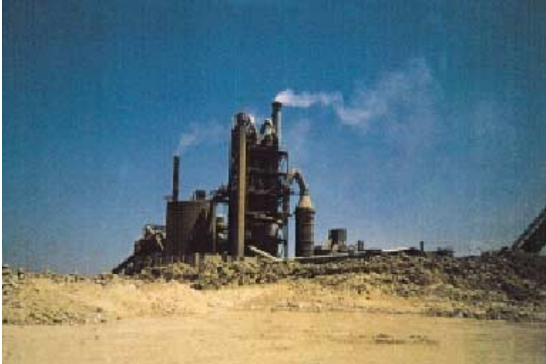
① Beni Suef cement plant
