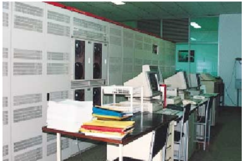
Digital switching system that switches and connects 6,000 subscriber lines
