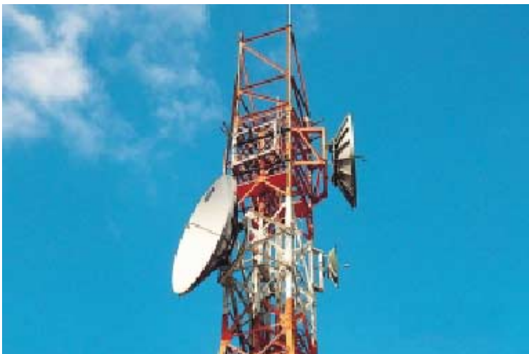
A parabolic antenna for transmitting microwave
