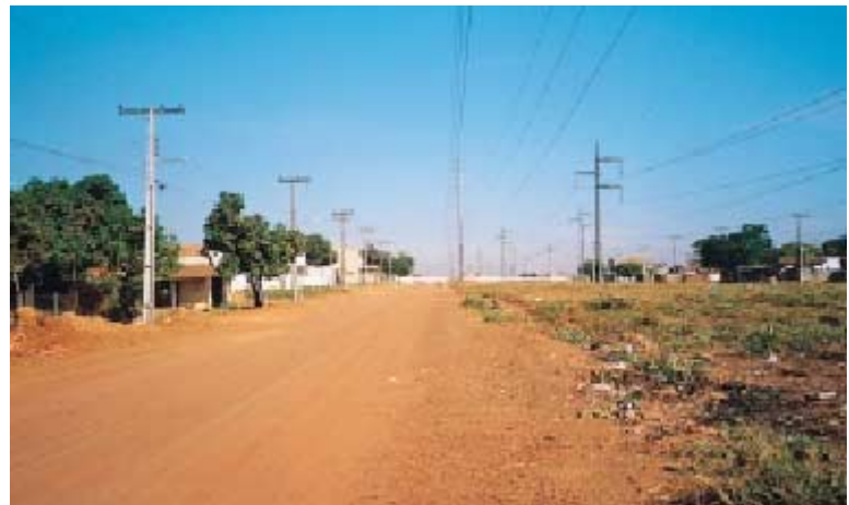
Constructed transmission lines
