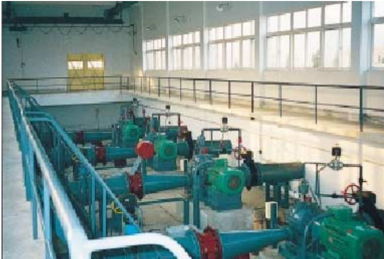
Pumping Station (Gaojiatai Water Treatment Plant)
