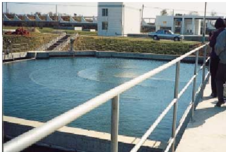
Oxidation Ditch/Half Turn Type (Sewage Treatment Plant)
