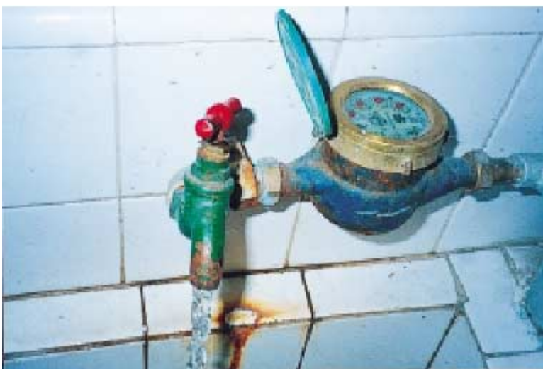
A water tap in a house of northern zone Meters are maintained in good condition.
