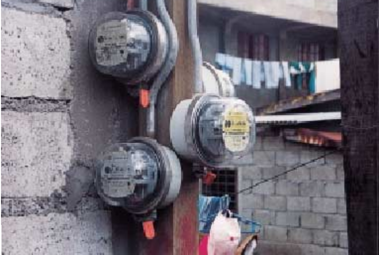
Meters installed by this project
