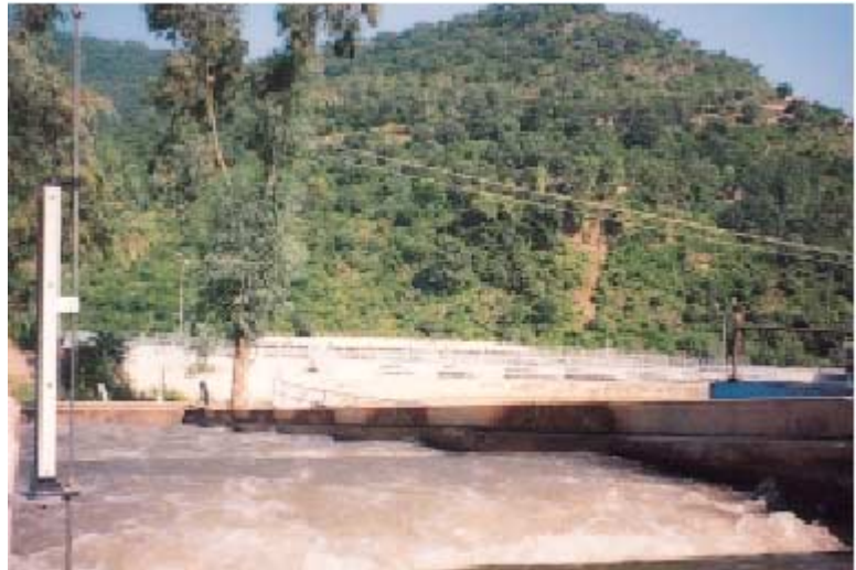
Simly Water Treatment Plant
