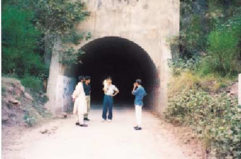
A tunnel under which the new and old conduction pipes are installed
