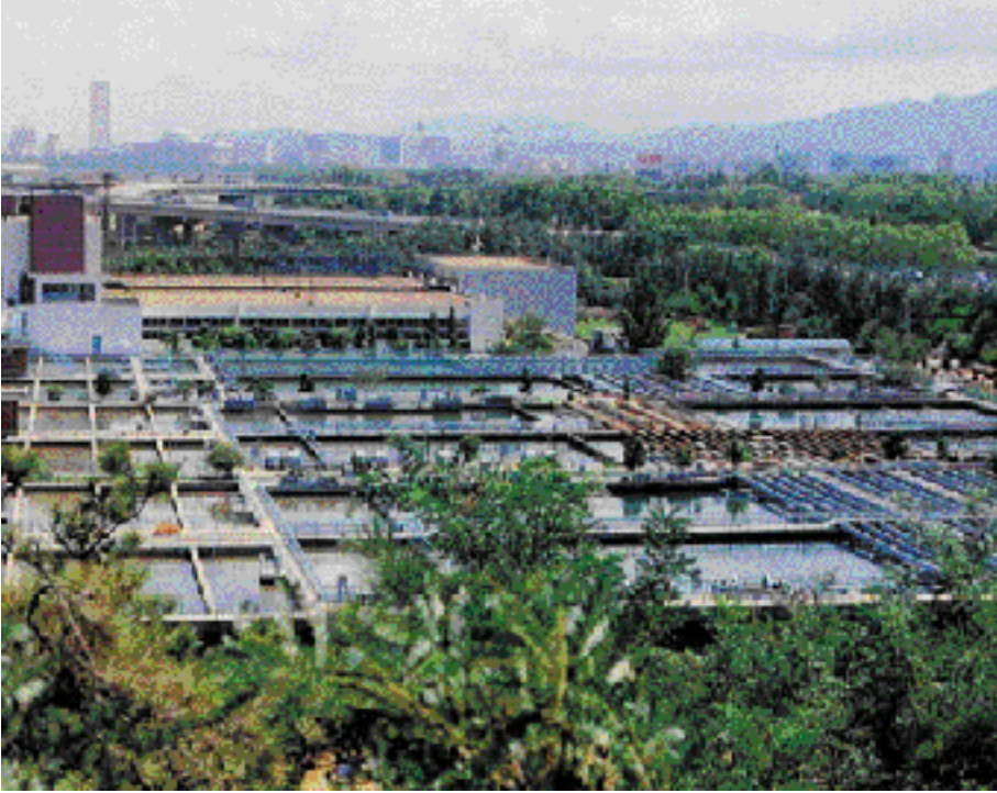
(1) Sedimentation Basin of the Parudan Water Source
