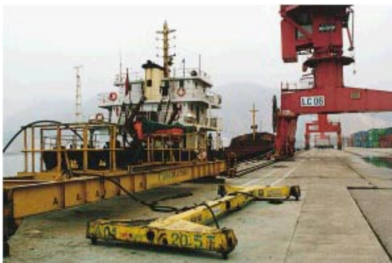
(2) Miscellaneous Cargo Berth in the Central Port Zone
