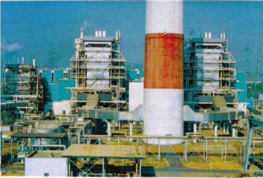
Power Generator (Left: Unit III, Right: Unit IV)
