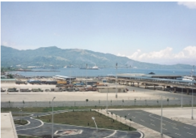
Batangas Port (Parking in the Port is now possible after its expansion)
