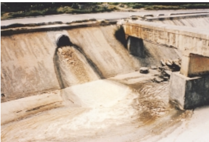
Sewage being discharged before the project in the Monterrey area
