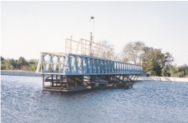
Secondary Sediment Facility of Noreste Water Treatment Plant
