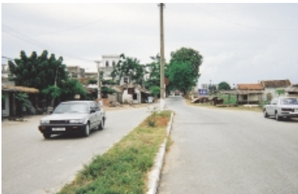
Widened Road in Ha Tay Province
