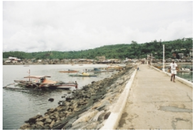
A Pier with Light installed by the City at Mauban Port
