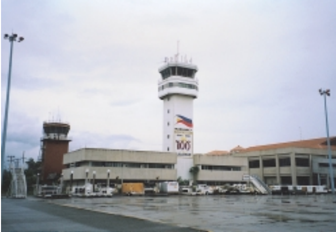
Control Tower at Mactan Airport
