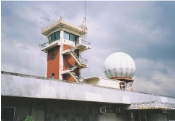
Radar Building (ARSRISSR)
