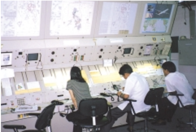
Control Tower : The Console in Sub-ACC
